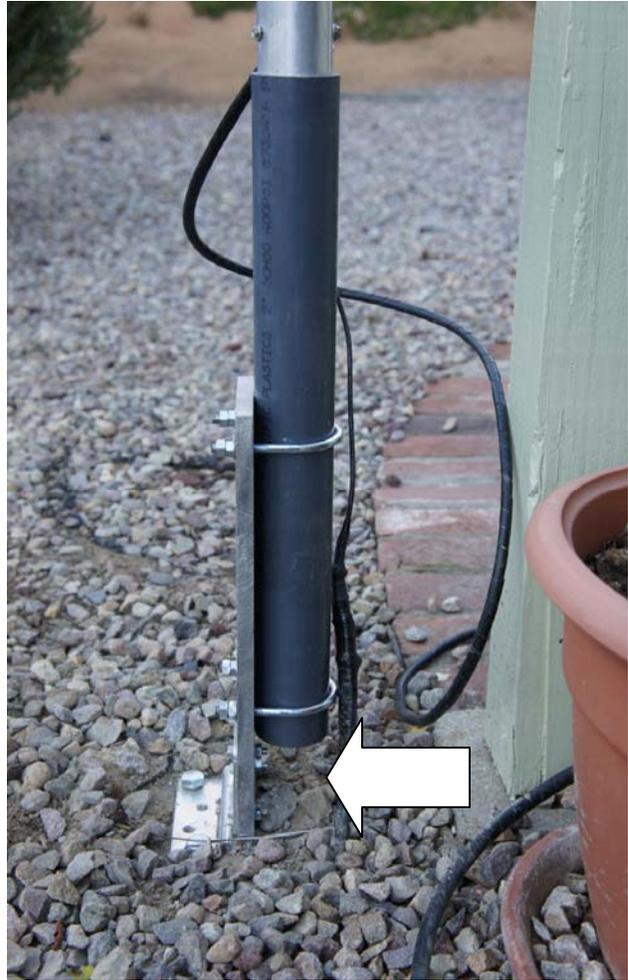
Note the gap between the bottom of the open tube insulator and the ground (arrow), to ensure rainwater can evacuate from inside the insulating PVC tube.
